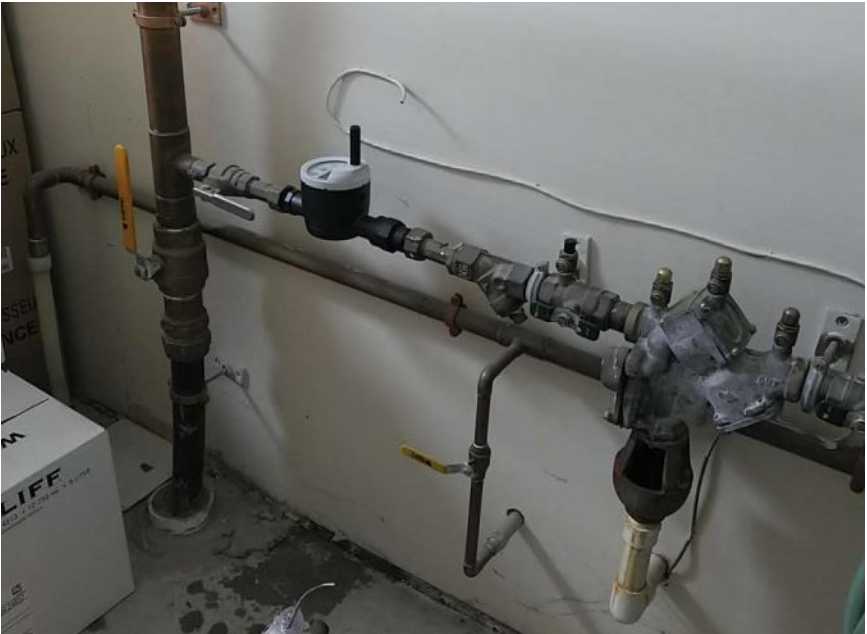
New meter install in a residential building.
