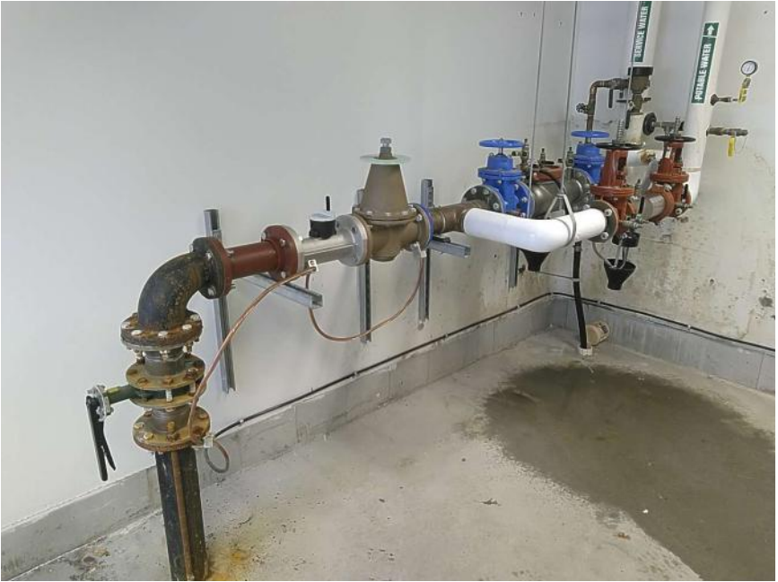
New meter installation in a commercial setting.
